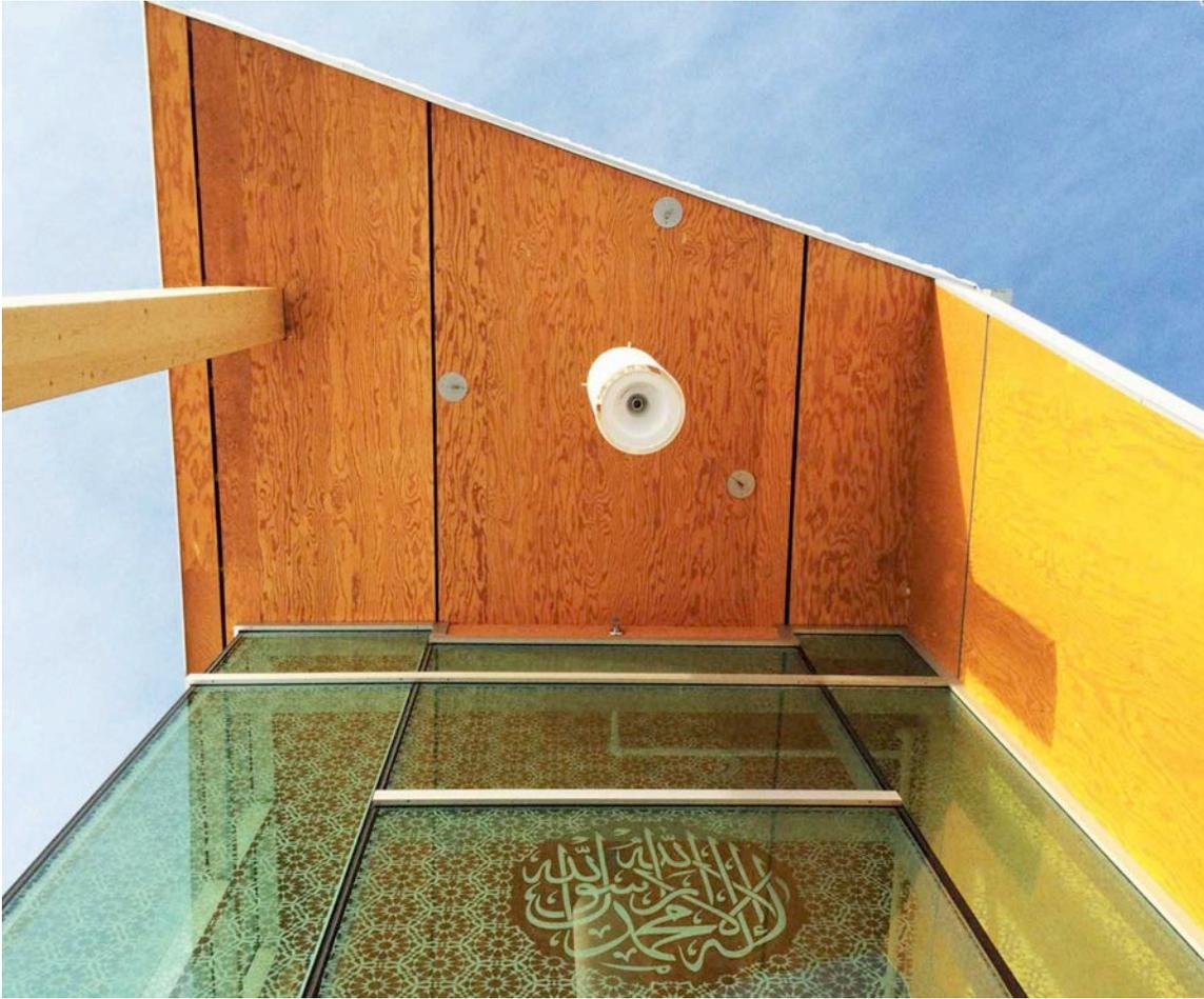
**Figure 3.** Detail of epigraphy and geometry sandblasted on glass above entry portal. Photograph by author, December 2016.
