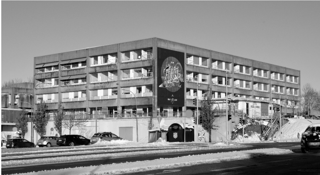
Figure 4: My workplace is at the top of the largest building of the abandoned former cultural center. Photograph: Exner
