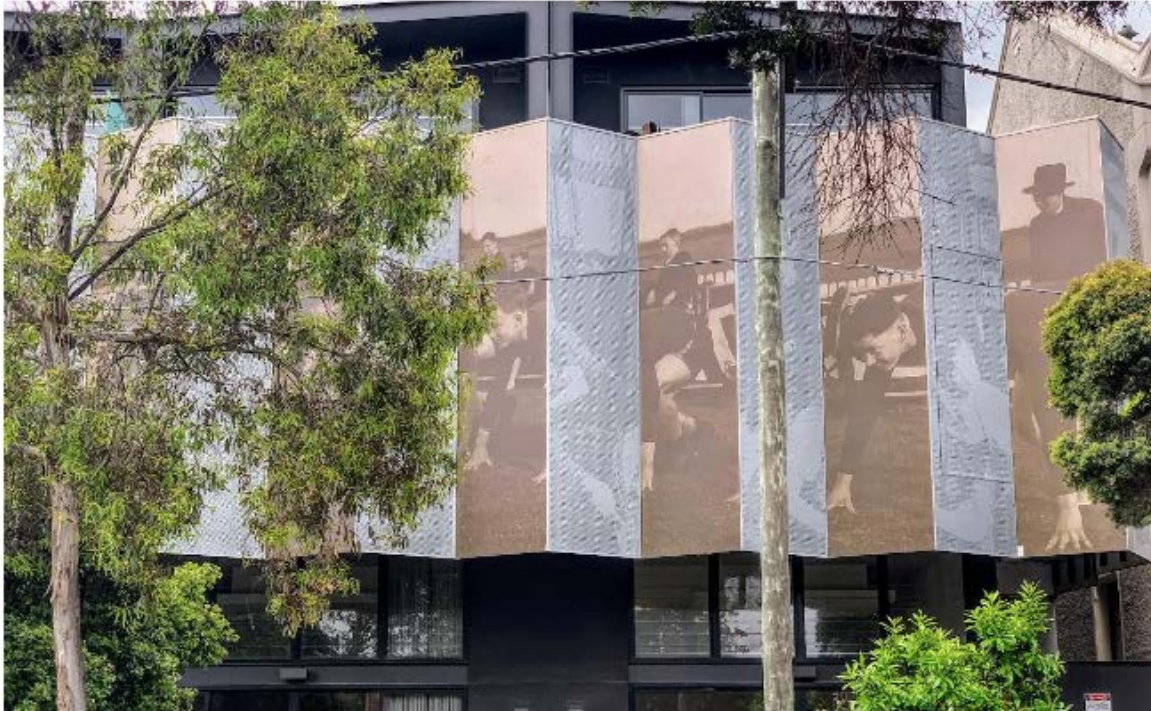
Fig. 3. Perforated screens on a new condominium development in Melbourne's Richmond harken back to the neighborhood's factories and mud-coated football grounds. Source: author.
