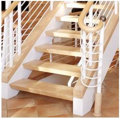
Figure 9. A newel post becomes an opportunity to celebrate the transition to ascending—with the help of the Metalworker, Woodworker, Metal Sculptor, and Stair Builder. Joe saved the day by making the end curves of the newel caps out of seventy-two laminations of maple. *Photo Credit: Omar Salinas*.
