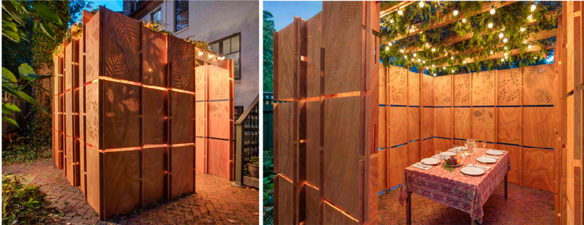
The interlocking panel construction and gaps between layers evoke the fragility of the desert hut with this “House of Cards” Sukkah, Chicago. Perforations in the forms of fruits associated with this holiday create a lantern effect at night. Amy Reichert Architecture + Design
