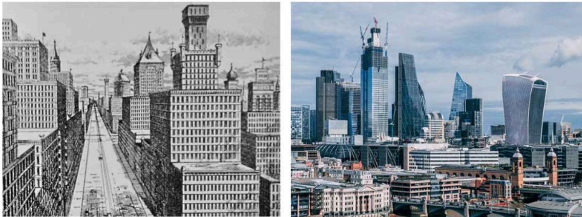
Fig. 4. Left: Proposal for North Mich. Ave. Chicago by architect Louis H. Sullivan office, c.1926, intended to encourage a common cornice height to promote a sense of continuity of the street as counter to the inevitable inclusion of high-rise towers in the wake of rapidly rising land values. Right: London's evolving skyline today, composed of disparate high-rise buildings unrelated to each other or to the historic urban fabric around them.
