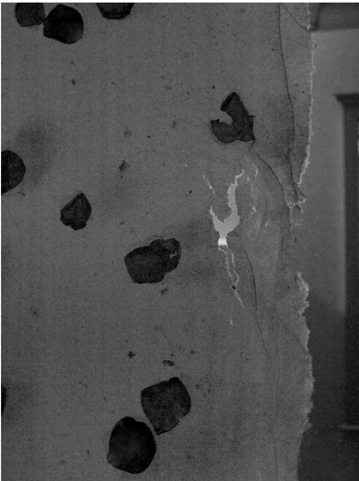
(above) detail of joints. All joints were modular pre-fabricated millboard discs which could adapt to any angle. By being a universal connection type, construction erection was simplified. Photo by M. Nicholas-Schmidt
