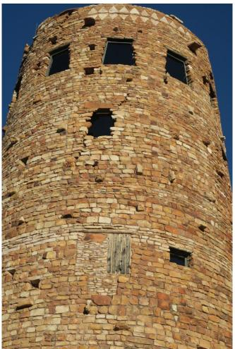
Fig. 1-4. Desert View Watchtower (detail). Note the surface texture, the deliberate cracks at the corners of the window, and the T-shaped opening filled with different materials, as if at a later time. (Linda Reeder, 2016)
