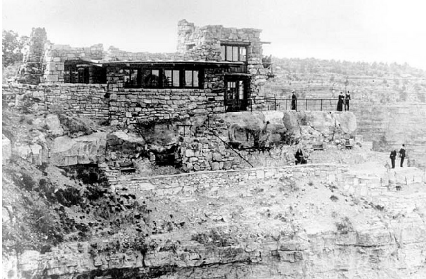
Fig. 3. East elevation of The Lookout with visitors viewing the canyon from different levels, c. 1915. (Fred Harvey, GRCA 11821, courtesy of NPS)
