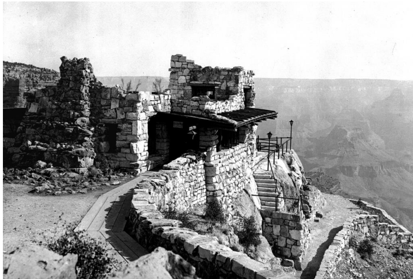
Fig. 2. South entrance to The Lookout, c. 1915. Note the plants growing on the roof. (Fred Harvey, GRCA 09722A, courtesy of NPS)
