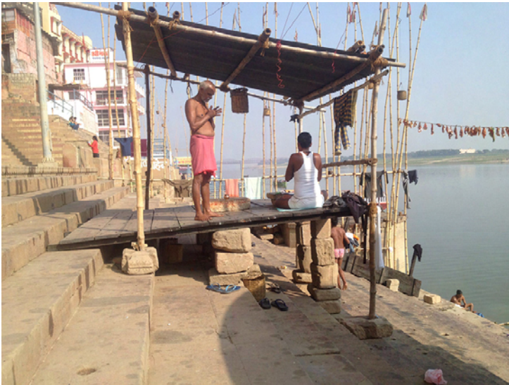
Figure 4. Shade structures on Panchganga Ghat
