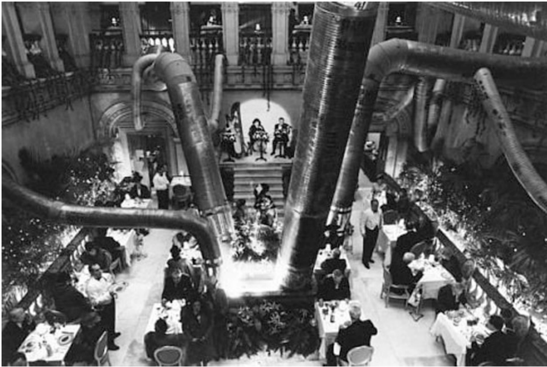
Fig. 3: The overbearing nature of a bureaucratic state out of control in Terry Gilliam's Brazil (1985) is expressed in the abundance of hideous ducts and pipes that dominate virtually every space in the film.
