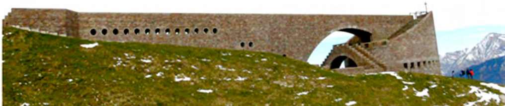
Fig. 1: Mario Botta's Chapel of St. Mary of the Angels, Monte Tamaro, Switzerland
