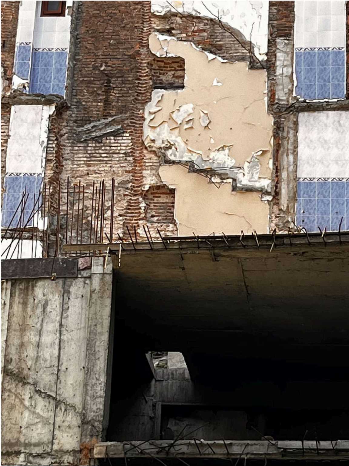
Figure 2: Detailed of textured masonry and ceramic wall remnants. (copyright belongs to Alison B. Snyder)
