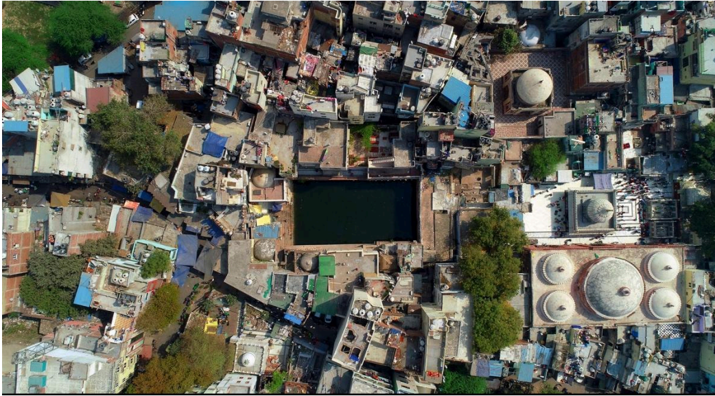
Figure 4: Aerial view of the Baoli and its dense historic urban setting. (Courtesy: Aga Khan Trust for Culture, New Delhi).
