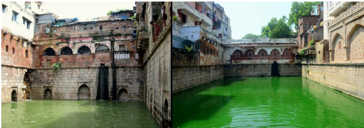
Figure 5: Conservation Intervention on the Baoli showing the Before (left) and After (right) scenarios. (Courtesy: Aga Khan Trust for Culture, New Delhi).
