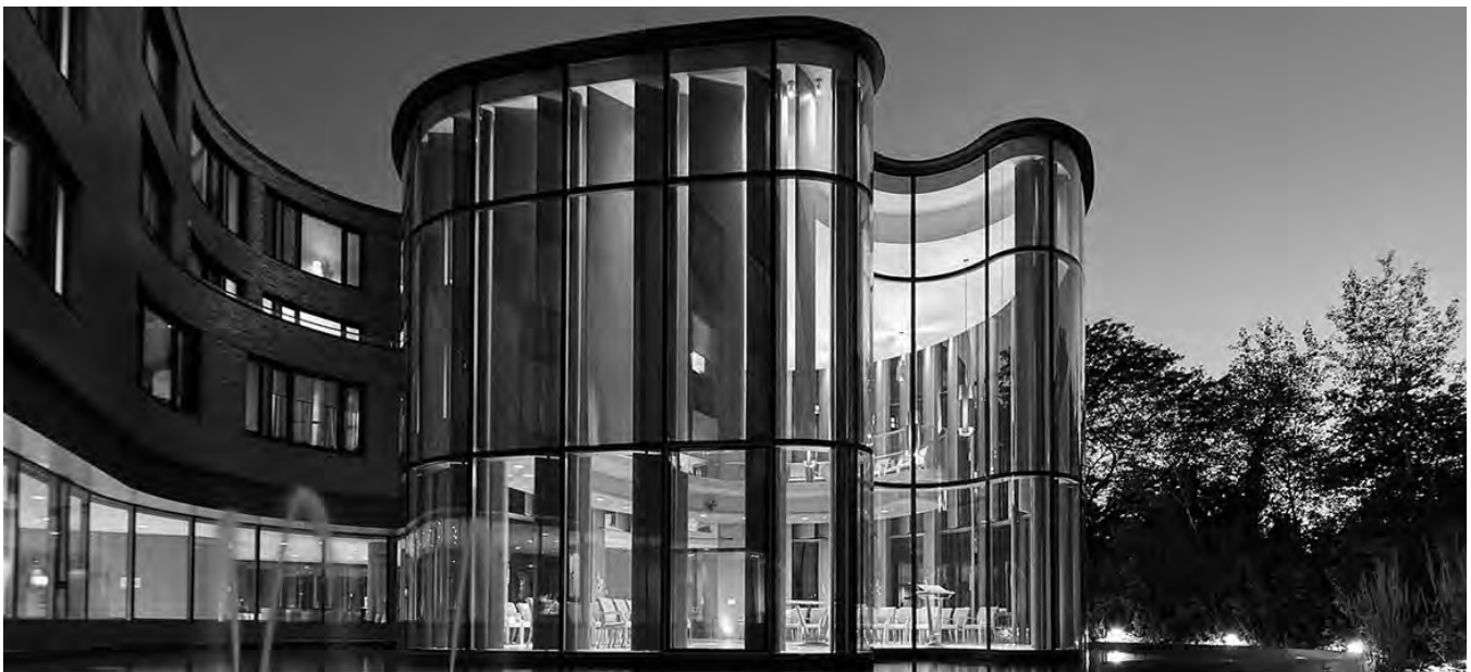
Sisters of St. Joseph, Toronto, Shim Surcliffe Architects
